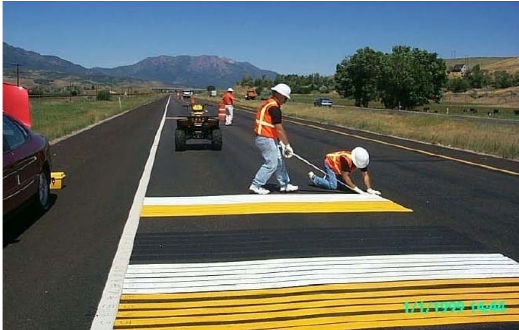
Figure 9 Applying the lines [35]
