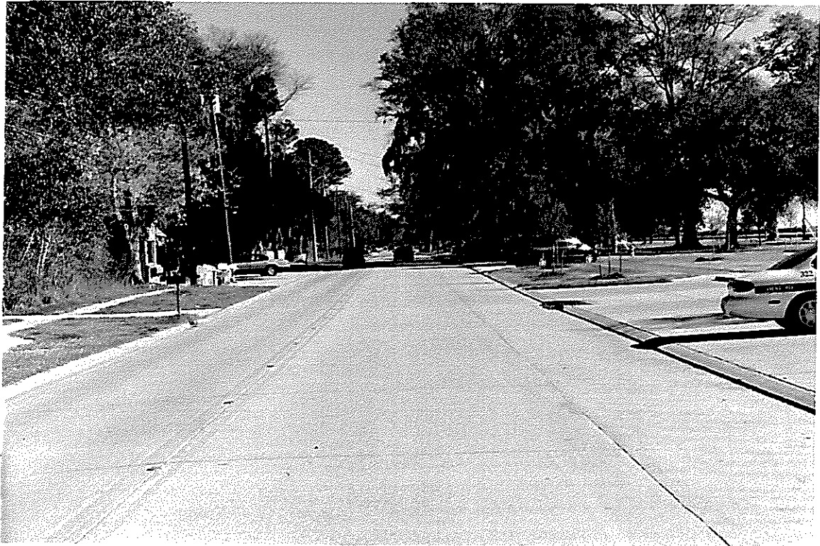
Figure 13 Completed project two years after construction
