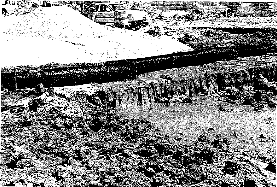
Figure 7 Excavation for repairs
