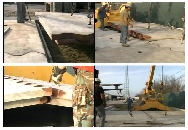
**Figure 16: Panel installation system**
