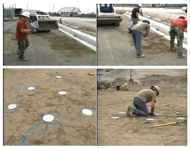
Figure 13: Sand layer placement and sensors
