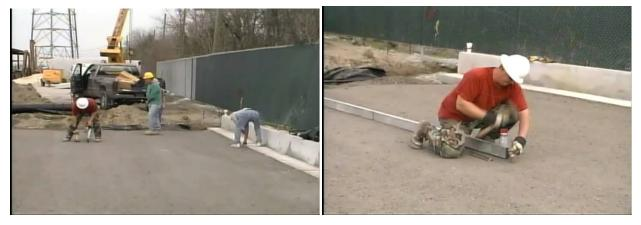
Figure 12: Slab layout on base course
