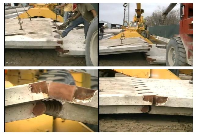
Figure 15: Longitudinal joint stitching
