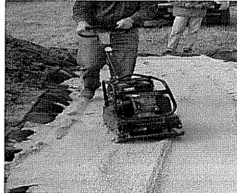
Figure 33 Compaction of trenches at PRF site
