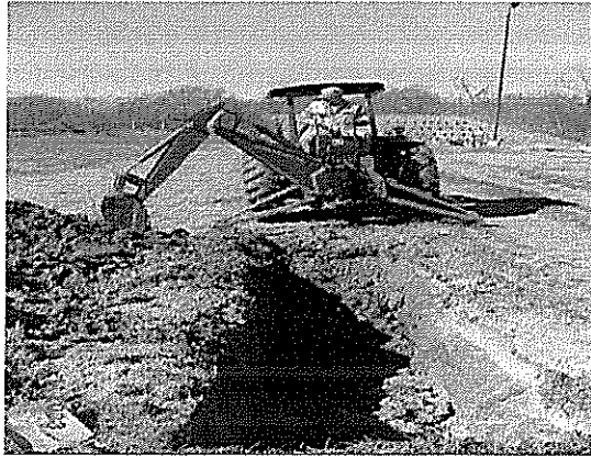
Figure 32 Construction of trenches at PRF site
