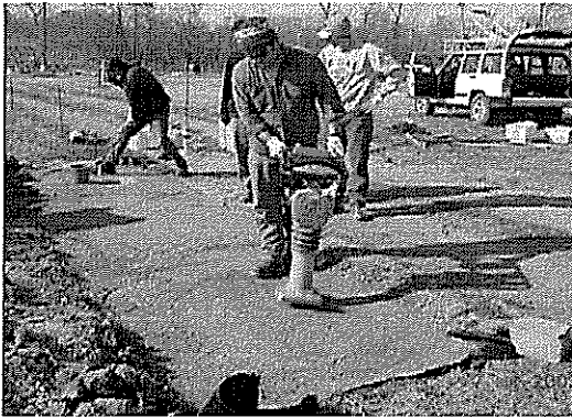
Figure 33 Compaction of trenches at PRF site
