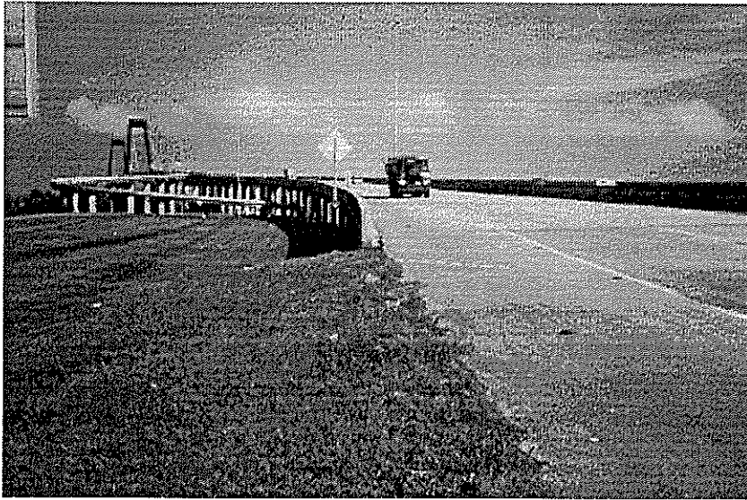
Figure 35 Site 5: Hale Boggs bridge south approach
