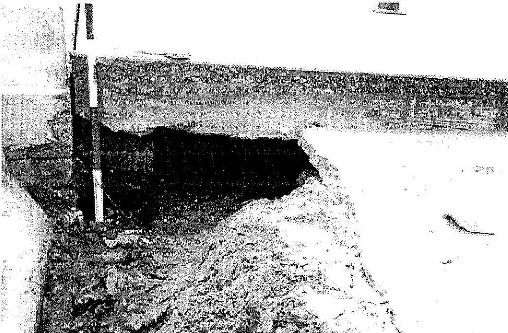
Figure 43 View of embankment under approach slab
