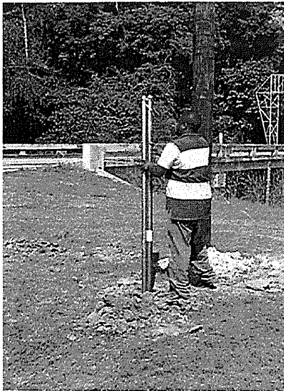
Figure 2 Technician installs copper grounding rods (Baton Rouge)
