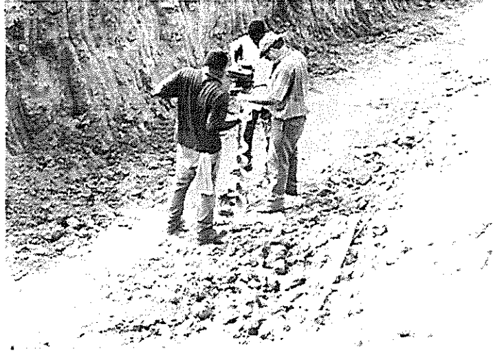
Figure 10 Manual digging of holes for installation of external anodes.
