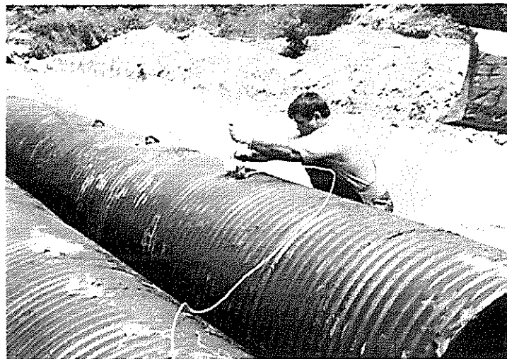
Figure 11 Electrical connection is being made to a section of culvert.
