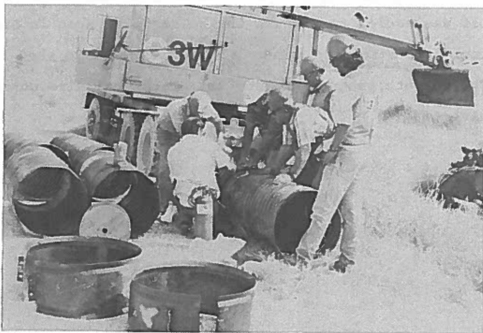
Figure 5. This is a culvert being prepared for installation.
