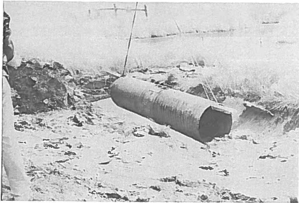
Figure 15. The unprotected culvert is lowered into the ditch.
