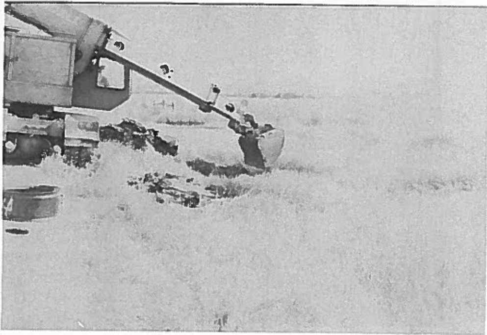
Figure 13. This is the unprotected site at the beginning of construction.
