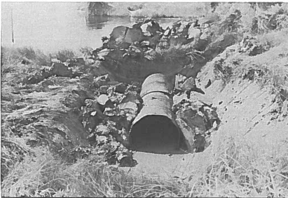
Figure 9. The culvert is being covered with the removed soil.
