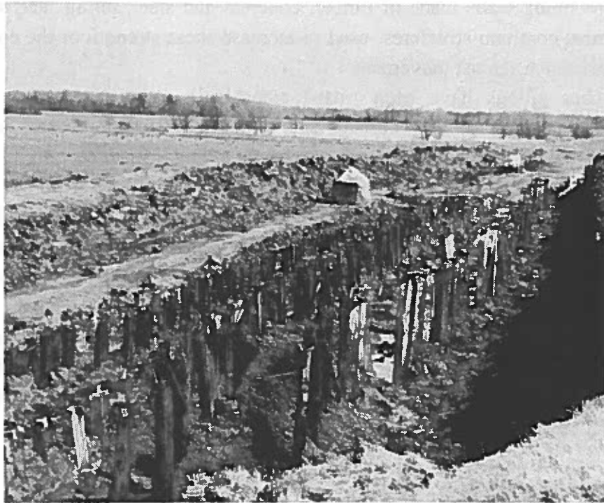
Figure 10. Unsuccessful attempt at stabilizing a failed slope by use of pilings at Chicago Mill site, Locality N17, northeast slope, Madison Parish, I-20 study area. Over 250 pilings were exposed in this one slope during repairs in 1987. The pilings do little to retard the movement of material that has a high shrink-swell clay content.
