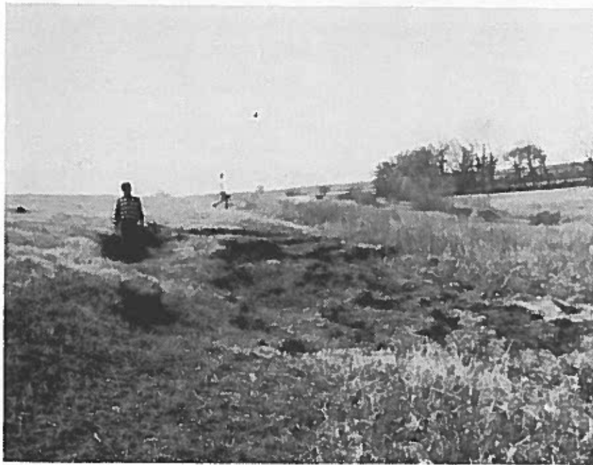
Figure 14. Slump exhibiting minor scarps caused by rotation. This failure appears on the northwest quadrant of Tallulah railroad site, Locality N18, Madison Parish, I-20 study area.
