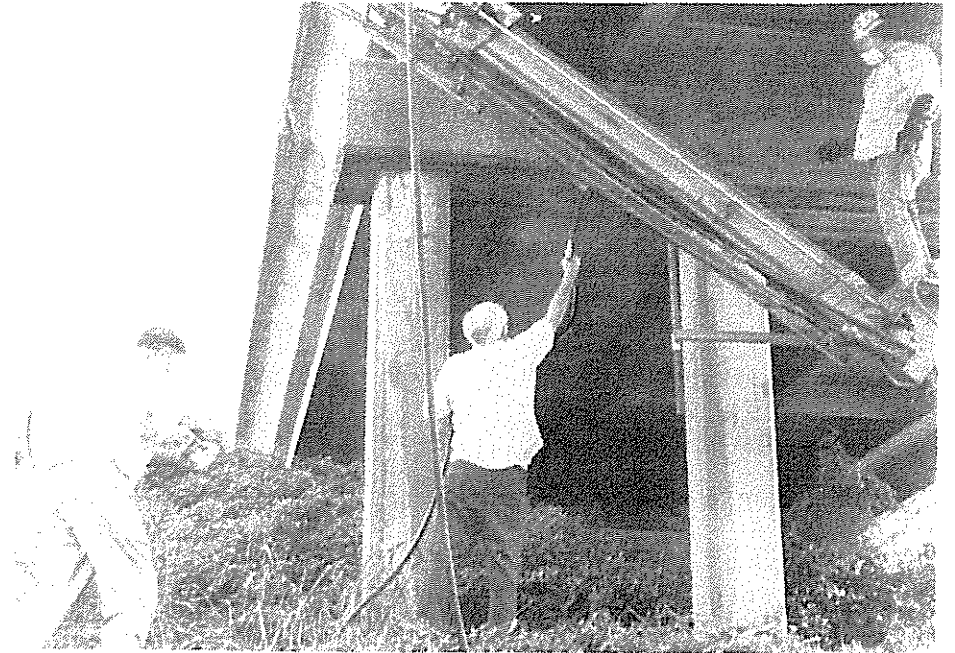
FIGURE 3 Treatment of the cap, Corey Overpass
