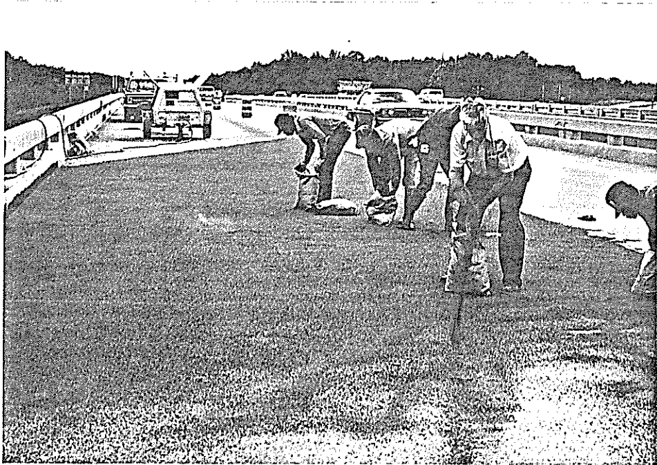
Broadcasting the Basalt Aggregate, First Coat
