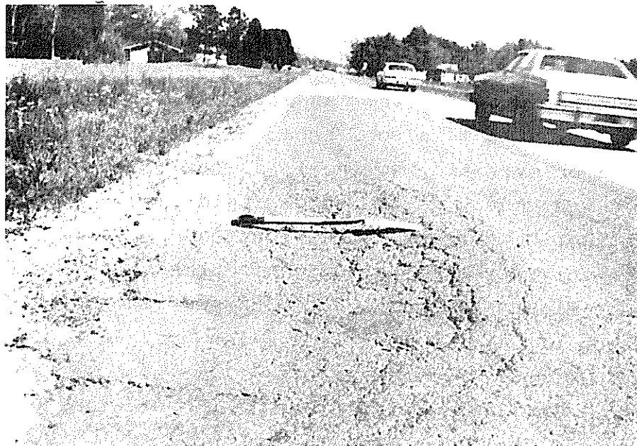
Rough Asphalt Test Section on La. 308 in South Louisiana
