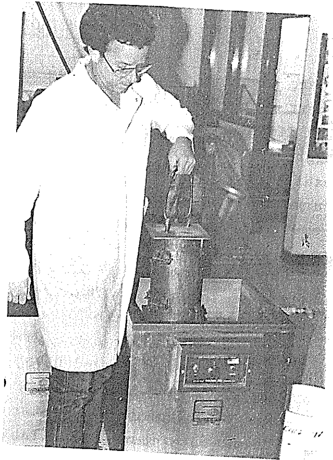
Placement of a Concrete Cylinder in the Curing Tank
