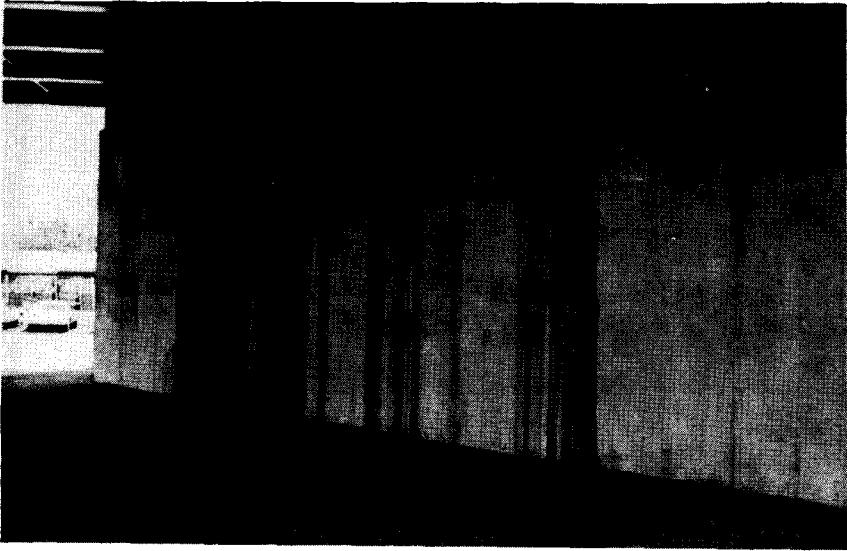
Aesthetically Displeasing Wall at Overpass
