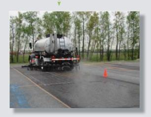
Asphalt tack coat is a light application of asphalt, usually asphalt diluted with water.
