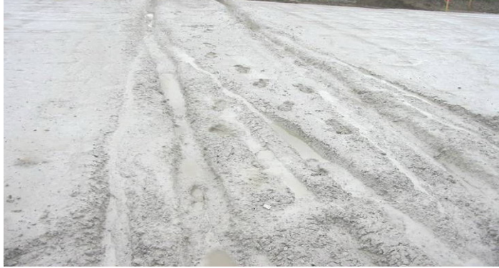
Figure 1 Pavement with a non-stabilized BCS base course
