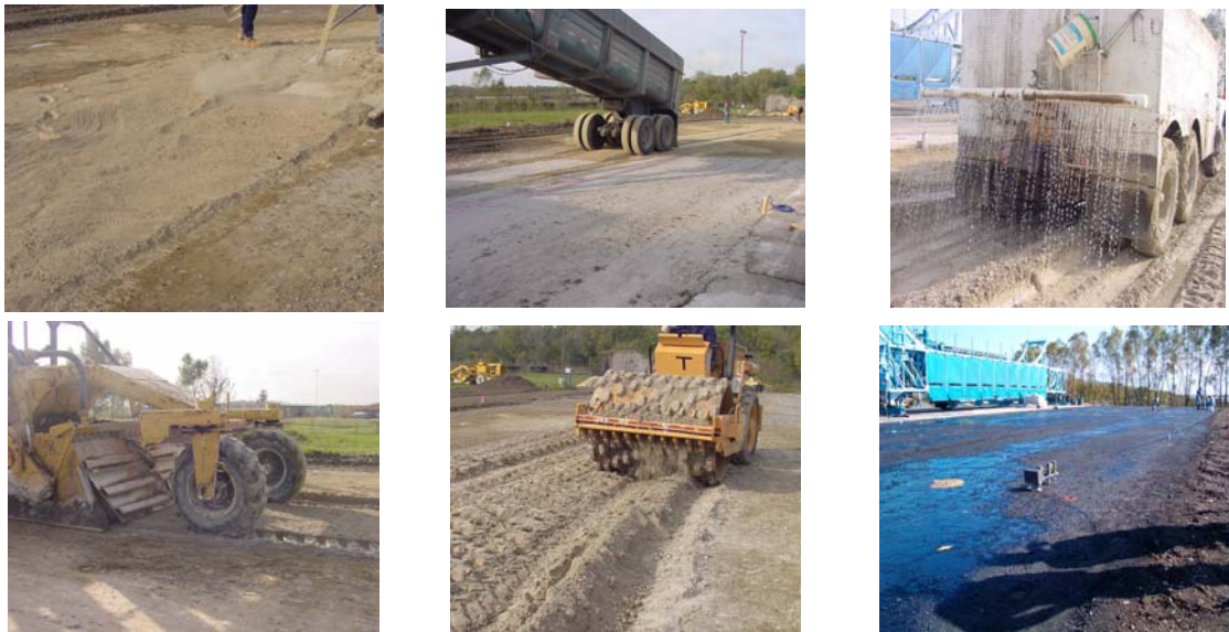
Figure 9 Photos of the stabilization process of BCS
