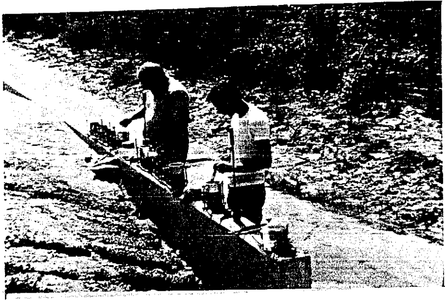
MOLDING SOIL-CEMENT SPECIMENS IN THE FIELD FIGURE 1
