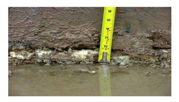
Figure 28 Polyurethane between slab and base course
